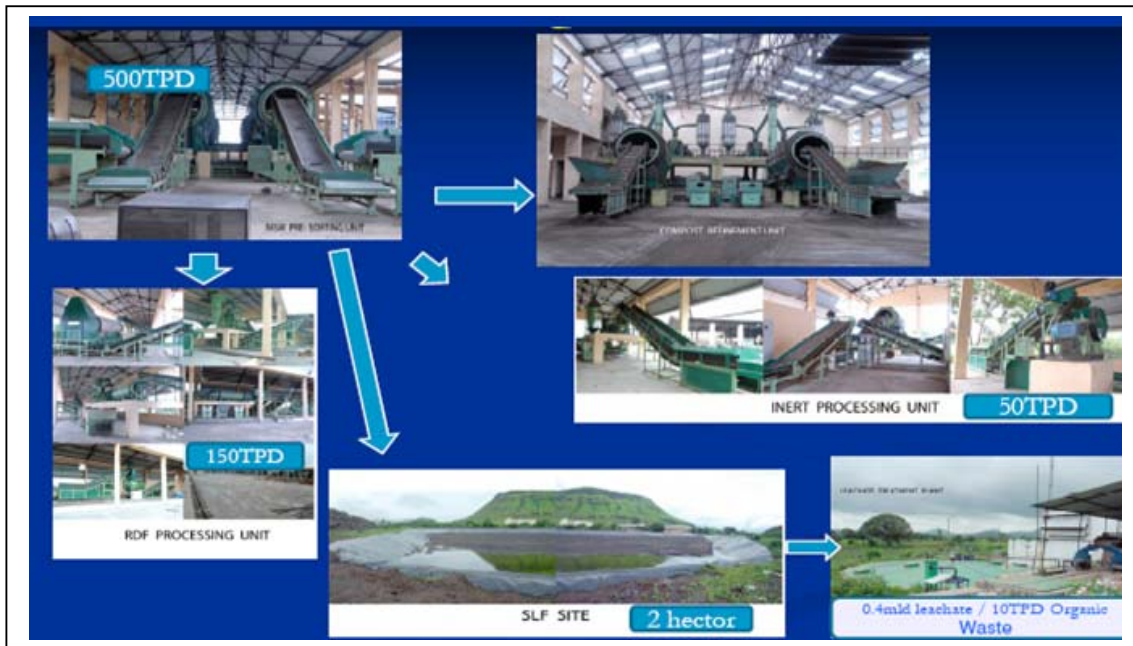
Figure 3.3 : MSW Treatment Plant and Sanitary Landfill Site at Khat Prakalp, Nashik
