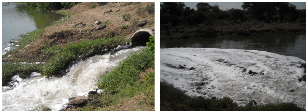
Treated Effluent with excessive foam released from Tapovan STP into River Godavari
