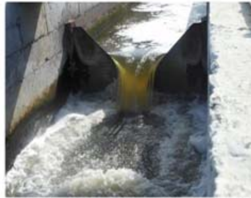
Treated effluent from Chehadi STP outlet with BOD more than permissible limit of 30 mg/L
