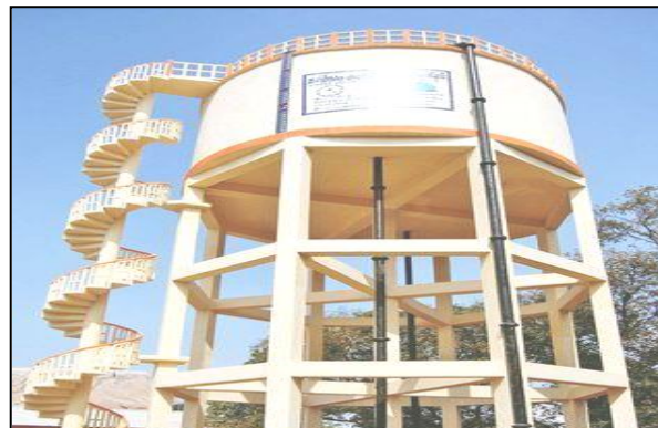
Water distribution tank
