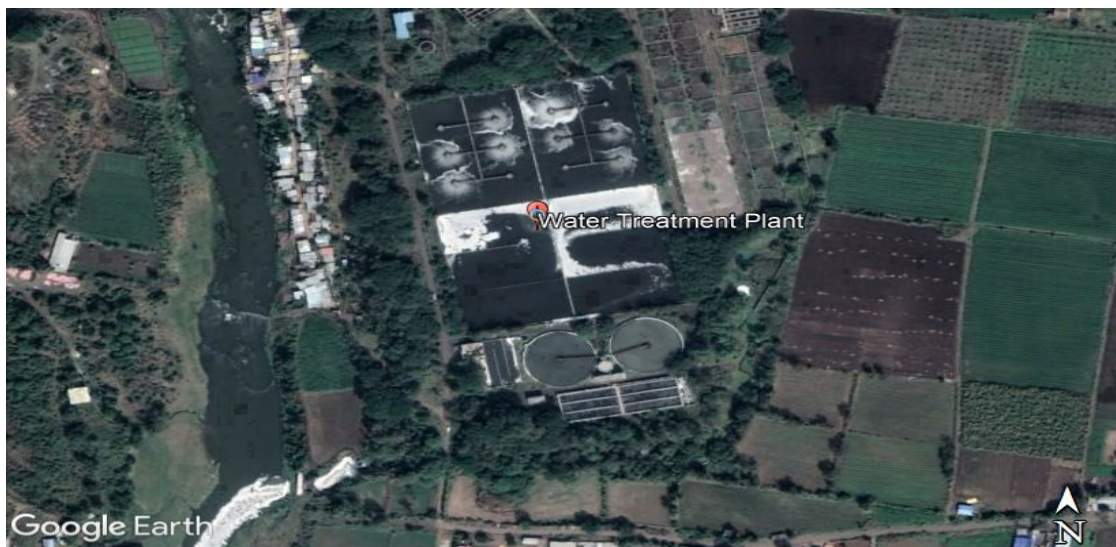
Fig 9.5 - Arial view of Water Treatment Plant
