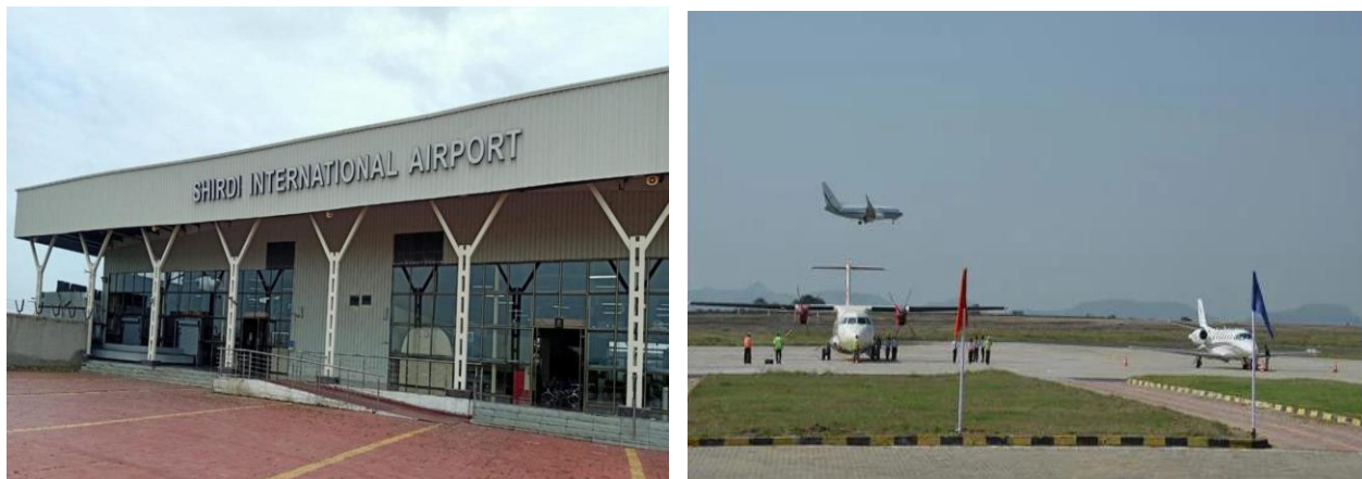
Fig 5.6 Airport facility at Shirdi
